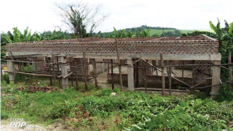
SACCO offices under construction
