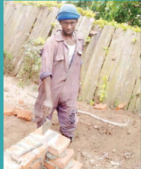
John Baptist at his construction work
