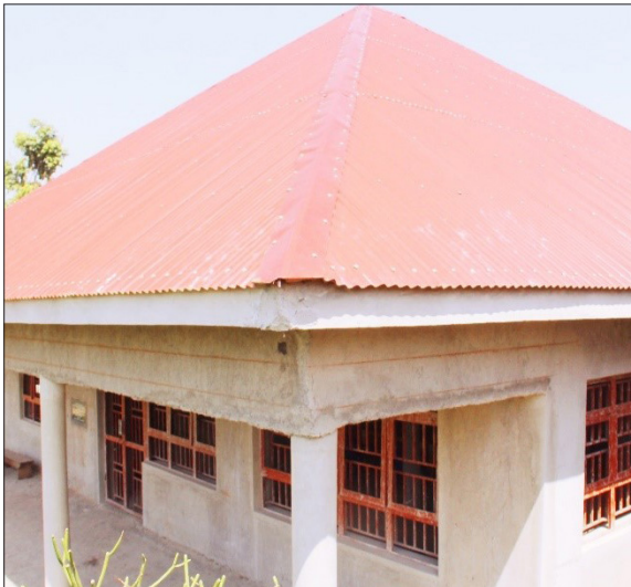
New SACCO premises still under construction
