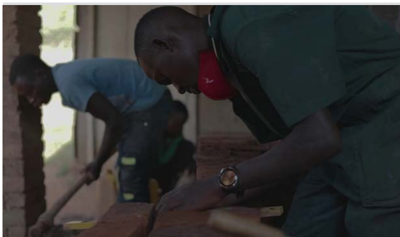
Students of brick laying and concrete practice during a practical lesson.
